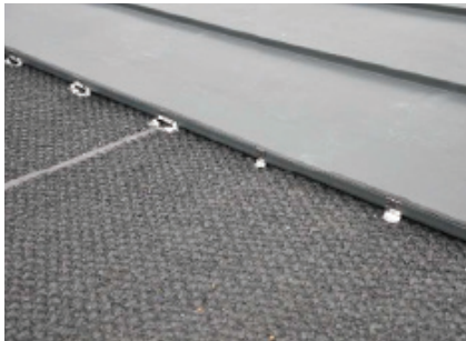
Example of using the METALDREN 450 g roofing foil under the KJG FALZ roof covering.
