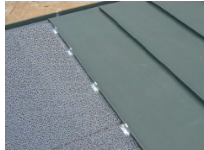
Example of using the structured mat MAT 8 mm under the roof covering KJG FALZ.
