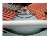
Polyester mat Enke-Polyflexvlies is a thermally bonded white colour mat with a weight of 110 g/m². Very good absorbency and ability to adapt to the unevenness of the base. Use with Enkryl, Enkopur, Enkepren as an insert that improves the mechanical properties of systems.
