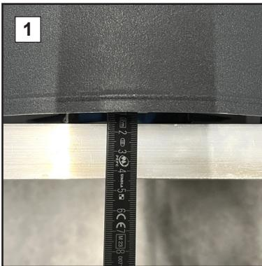
The top cover of the ridge cap must overhang by approximately 15 mm.
