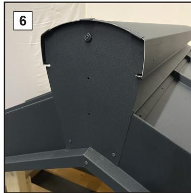
Detail of the correct installation of the front ridge cap ending UNI.
